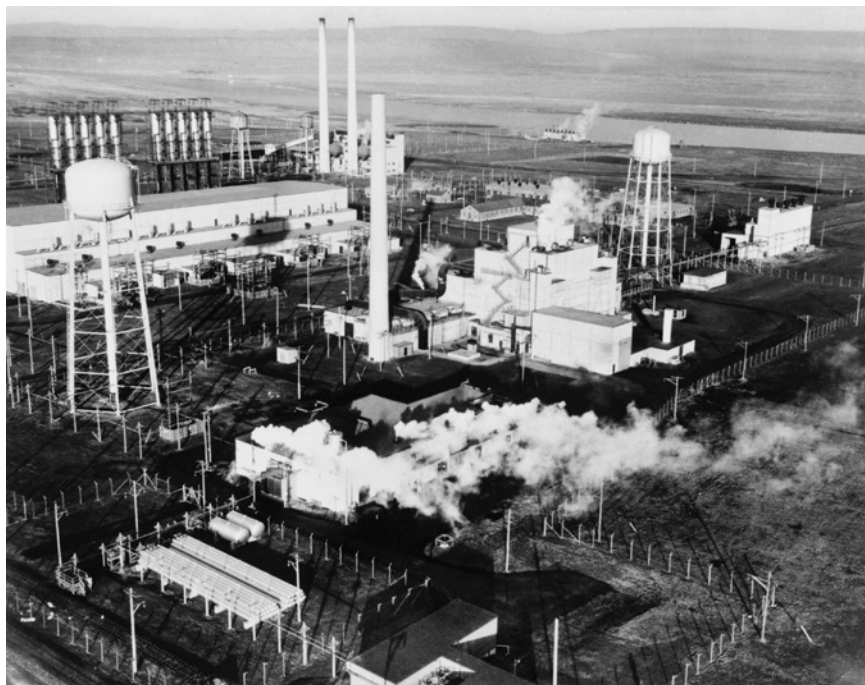
FIGURE 6.4 Aerial view of the 100-B Area of the Hanford Site, showing reactor B, the first large-scale nuclear reactor ever built. This produced plutonium-239 for the second atomic bomb which was dropped on Nagasaki.
